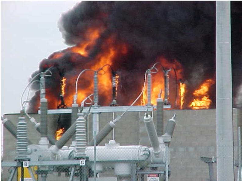
The trigger event was a short circuit fault on a 220/30 kV transformer. The circuit breaker failed to open and the fault was cleared by Zone 2 distance protection. After the short circuit was cleared, a severe transient arose creating instability between the Western and Eastern regions. The two sections split and islanded, eventually losing generation and leading to partial shut down.
