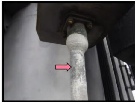
Photo 7: Yard, ground floor, external, 33 kV feeders, residue to cables - Positive Asbestos Debris
